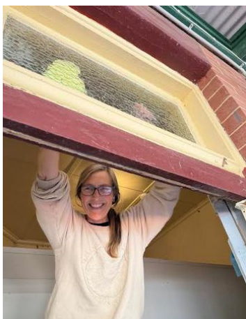
Lyndall busy removing paint from a window
